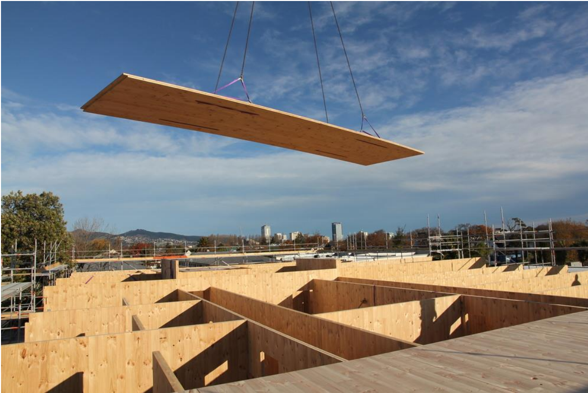
Cross Laminated Timber (CLT) structural building panels are being used for floors, roofs and walls in commercial and residential buildings. Source: XLam Australia
