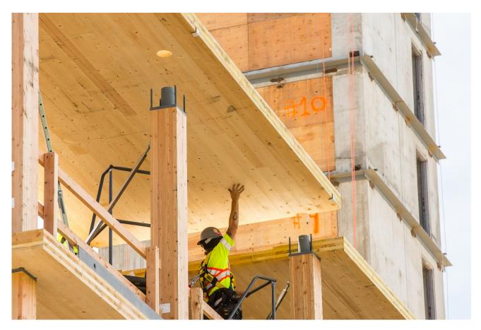
CLT Mass Timber Construction is factory-profiled for rapid assembly on site. Proposed changes to New Zealand building law that recognise prefabrication as a means of achieving quality and efficiency are exactly in line with the aims of Mass Timber construction.
